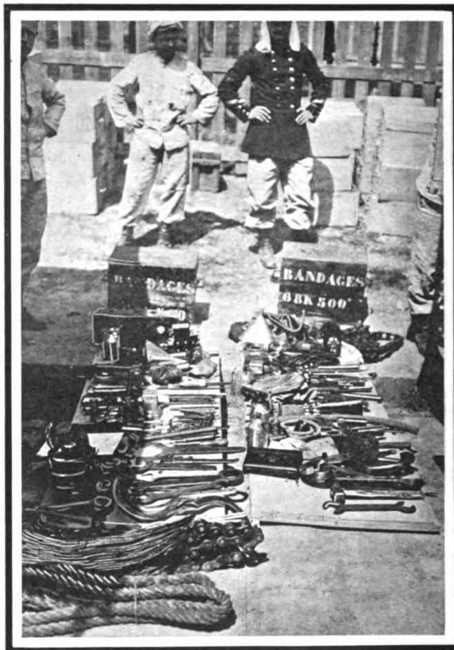
Spare parts of two cars laid out for inspection
